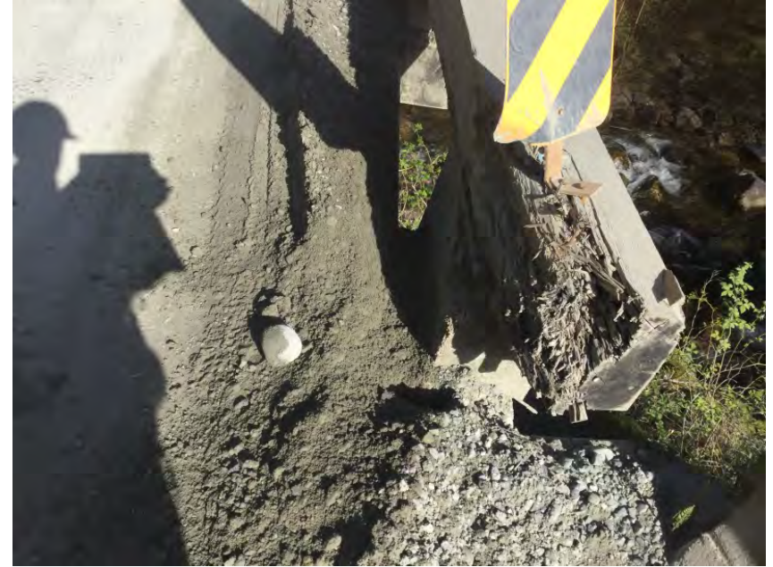
Damaged guardrail
