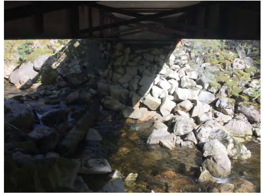
Left Bank Abutment when facing downstream
