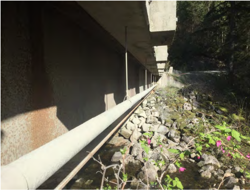
Utility on underside of deck
