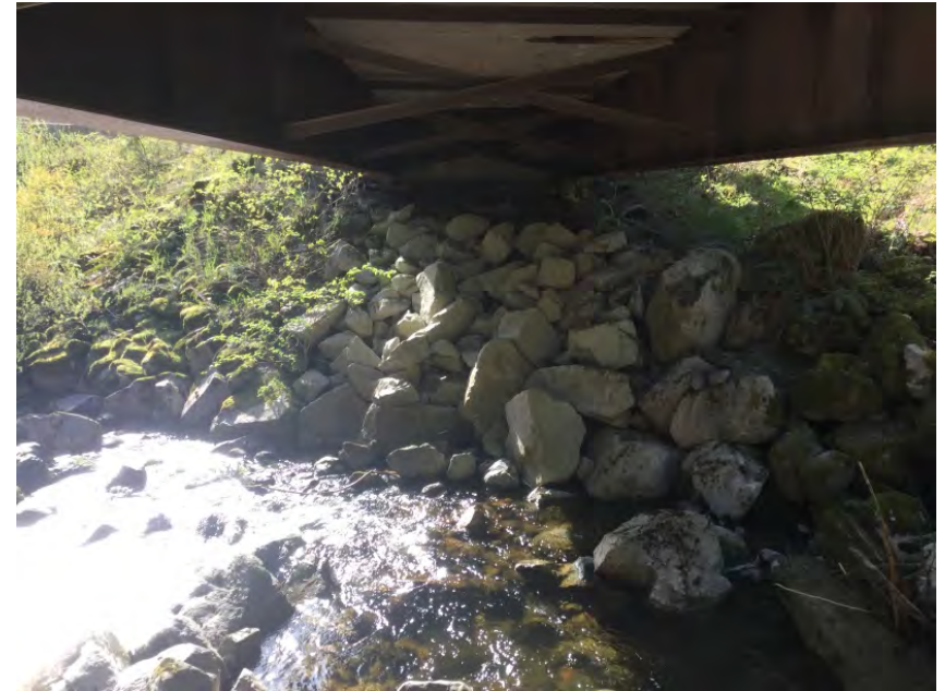
Right Bank Abutment when facing downstream
