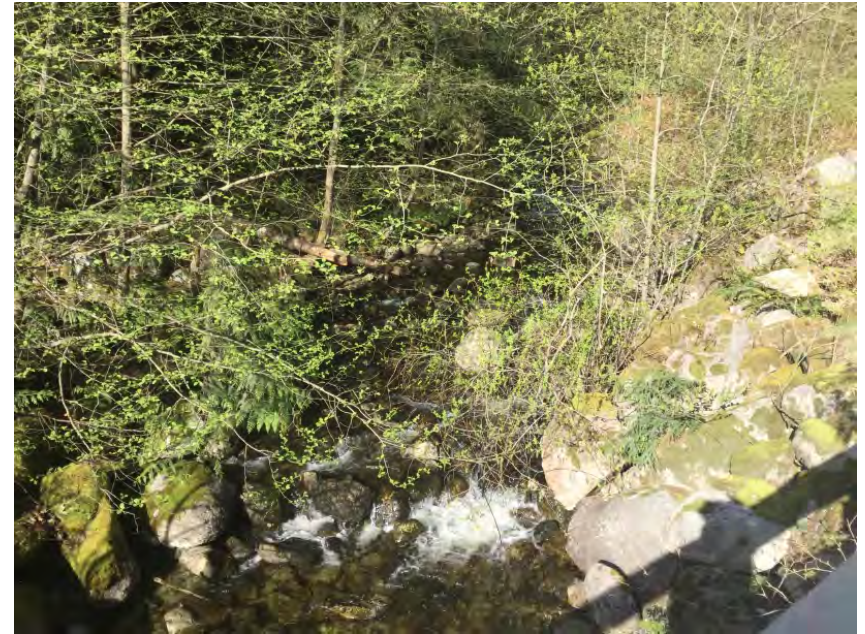
Looking upstream from deck
